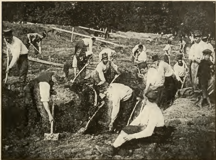
BELGIANS DIGGING TRENCHES
